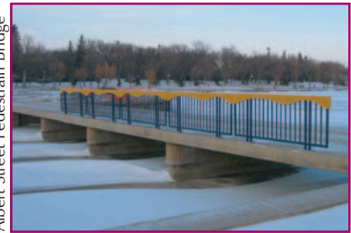
Albert Street Pedestrian Bridge
