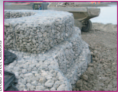
Broad Street Gabions
