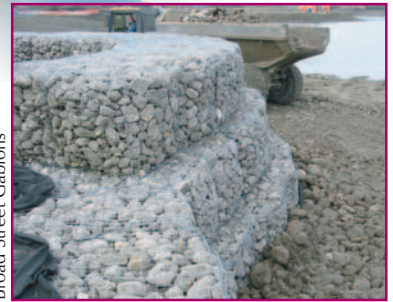
Broad Street Gabions
