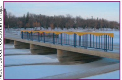
Albert Street Pedestrian Bridge
